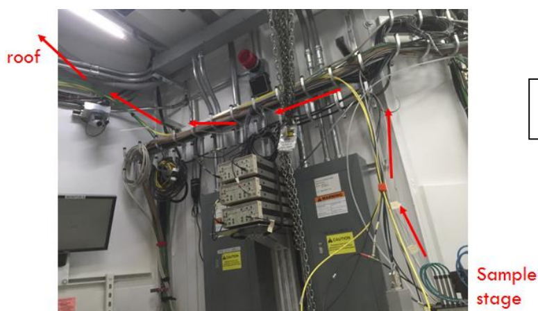
Fig. 4 Membrane gas tubing in 13BMC
